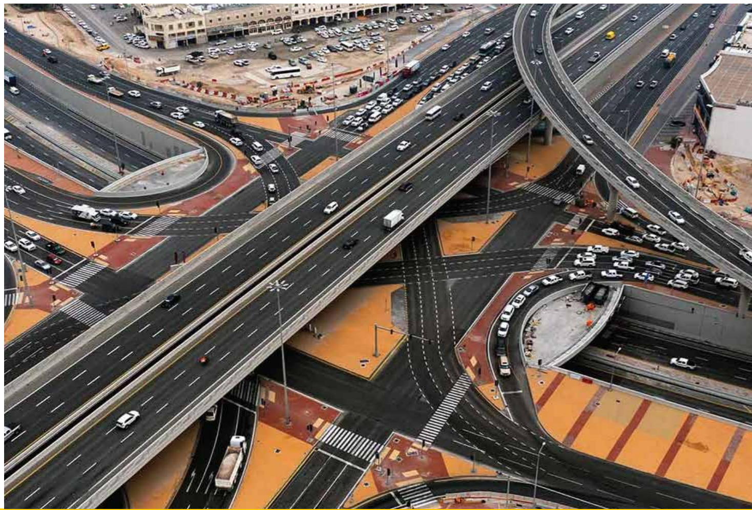
MUBAIREK BRIDGE DOHA, QATAR
