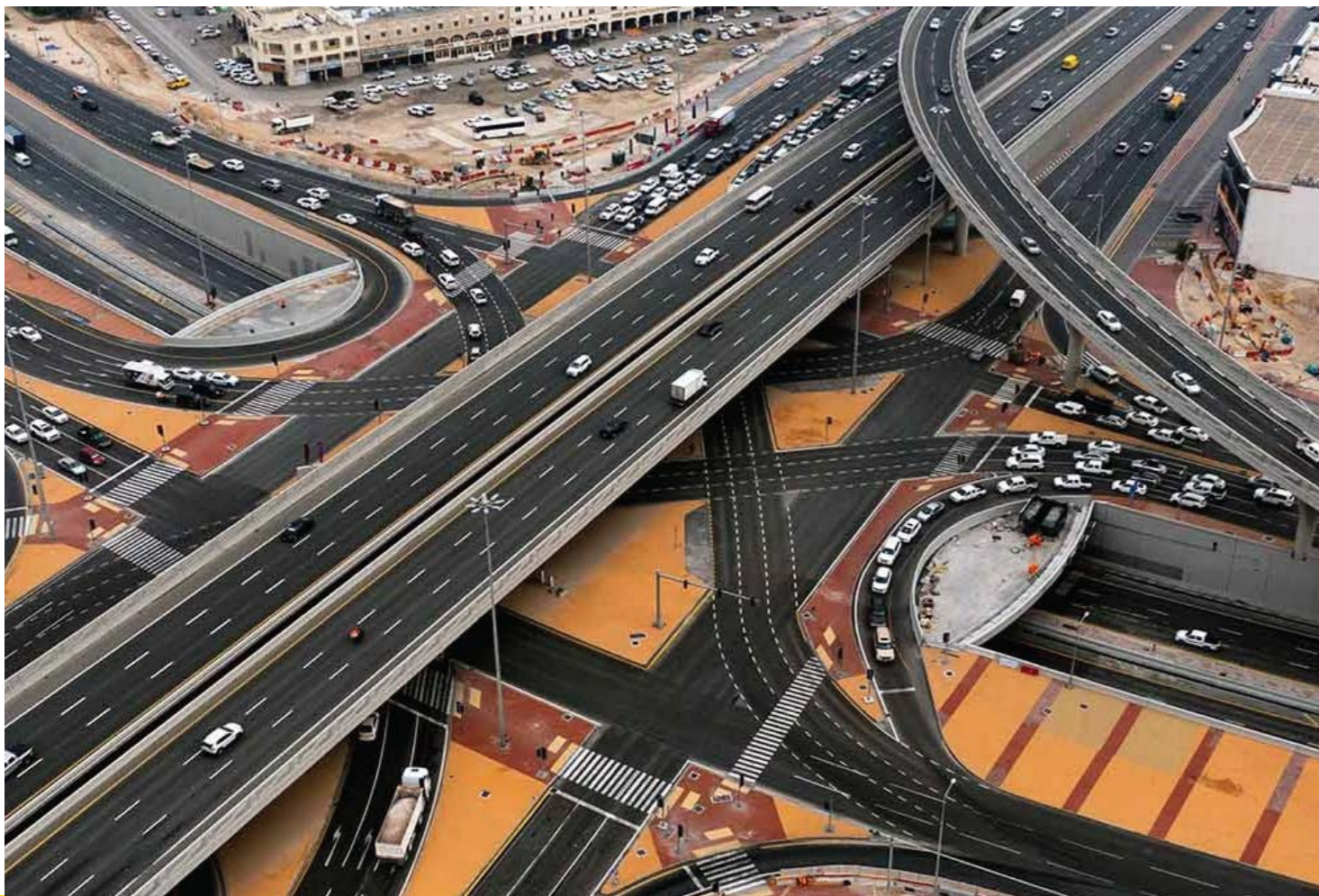
MUBAIREK BRIDGE DOHA, QATAR
