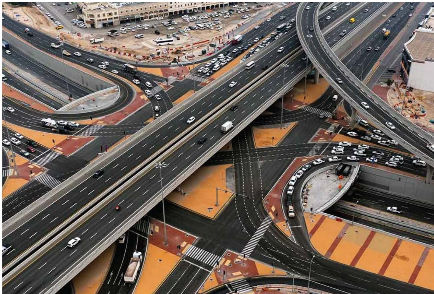
MUBAIREK BRIDGE DOHA, QATAR
