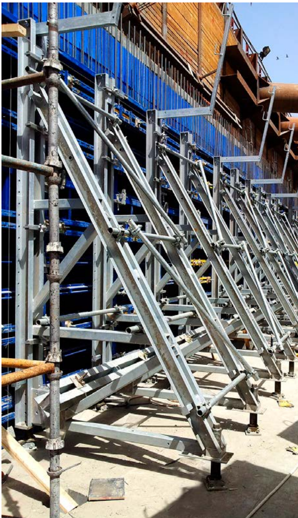
Modular supporting unit formed by combing Attachable frames 1.50 m
